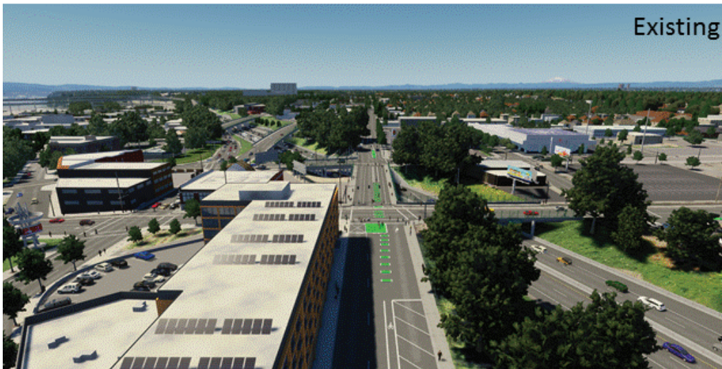
Figure 2-5. Broadway/Weidler/Williams and Vancouver/Hancock Highway Covers (Existing and Build Alternative)
